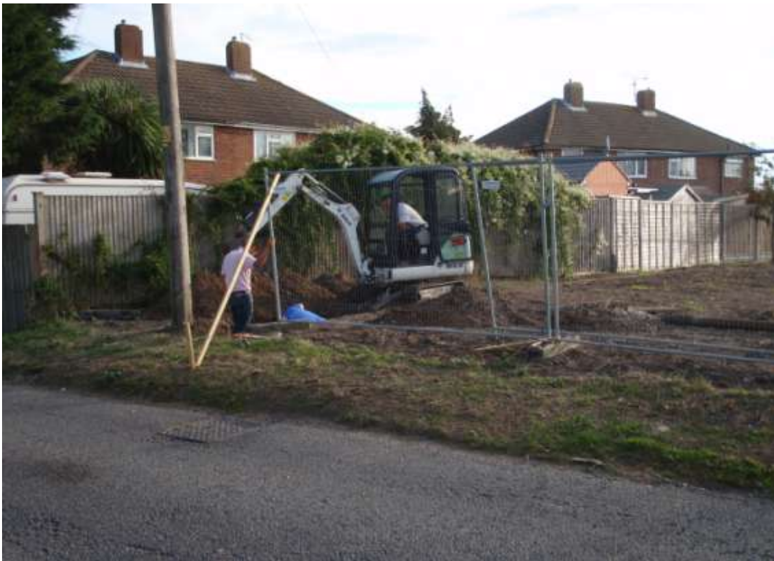
Plate 3. View of the drain being connected (looking north-east)
