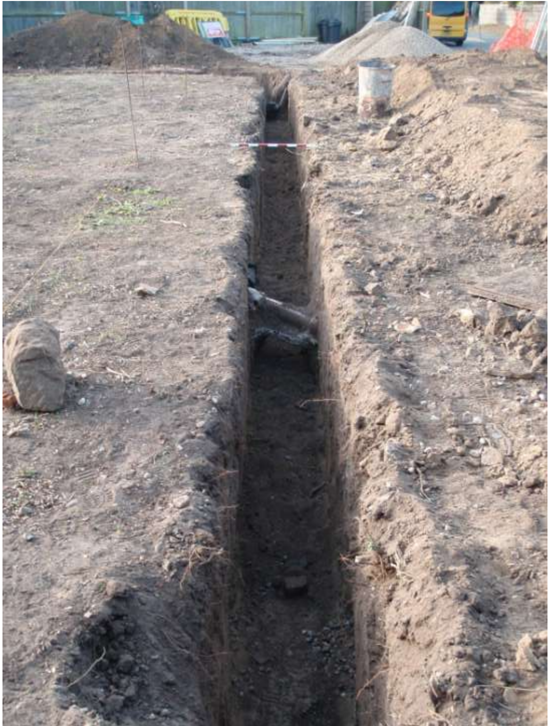
Plate 4. View of the drainage trench (looking east)
