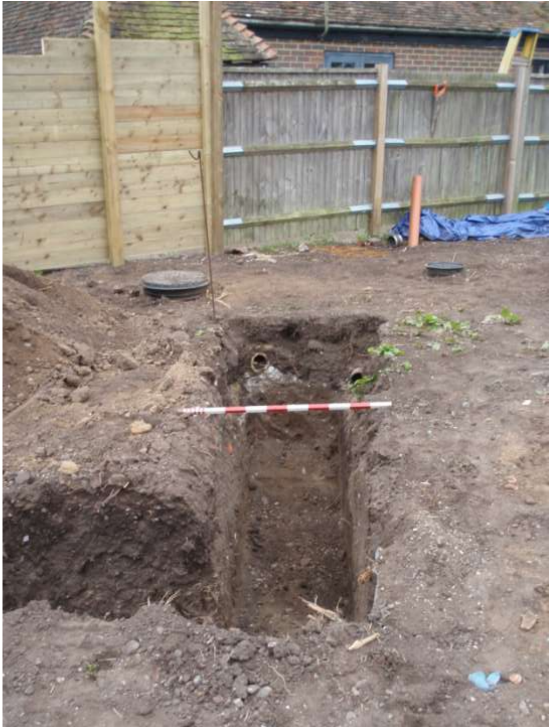
Plate 5. View of the drainage connection to proposed houses (looking north-west)
