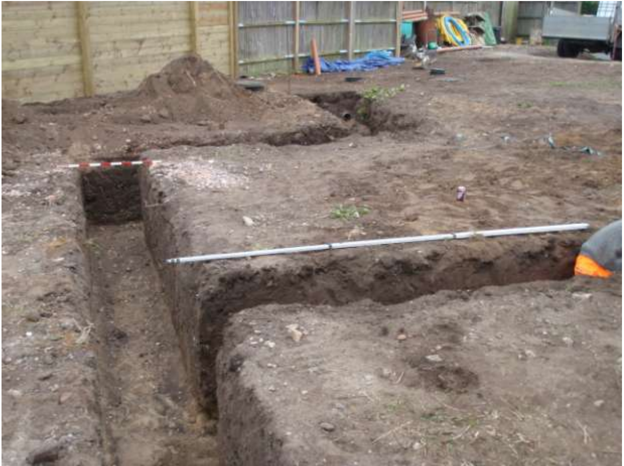
Plate 6. Cutting of the foundation trenches on north-west side (looking north)
